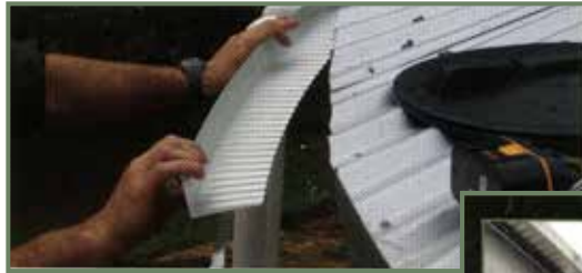
Fitting of gutter system
